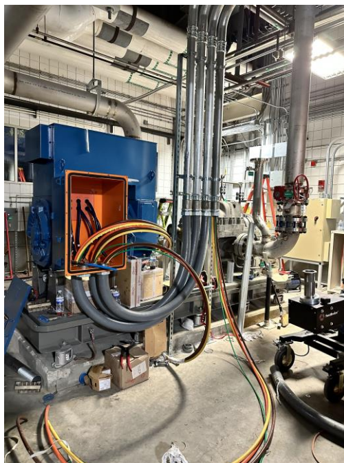
Figure 2.3.3. Magnet cooling water pump MCP1F shown during the connection of electrical services from the variable speed drive.
