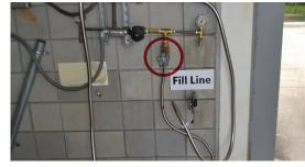
2 Identify the liquid (fill) line on the wall.
