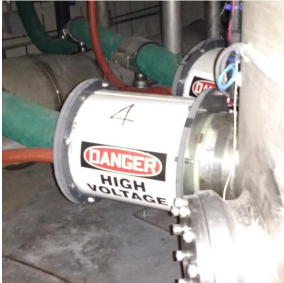
Figure 2: The cable-to-magnet terminals are covered with insulating cable covers to shield personnel from exposed conductors.
