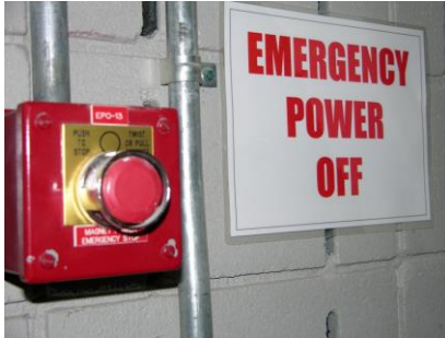
Figure 8: Wall-mounted Emergency Power Off button. EPO buttons are located near the exit of each magnet cell in the DC Magnet Building.
