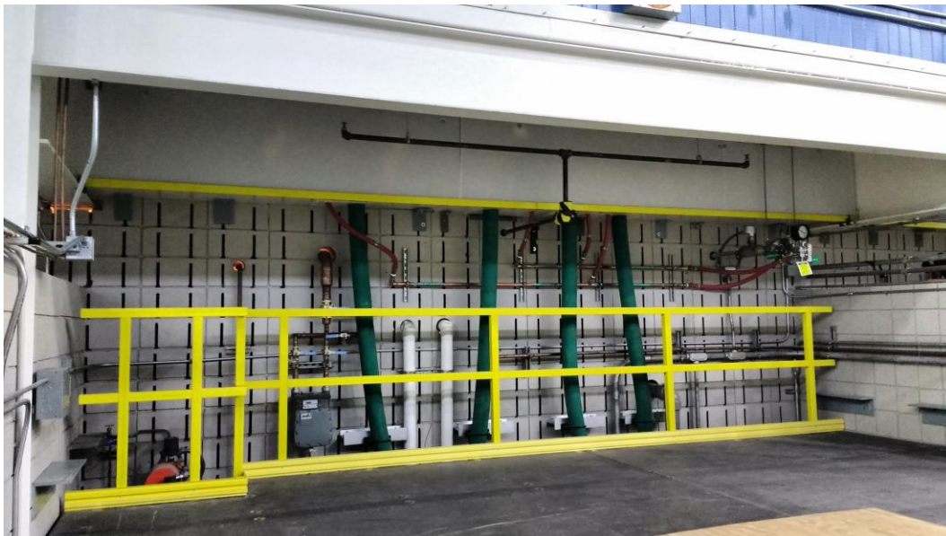
Figure 1: Green, water-cooled cables connect to the power supply bussing at the back wall of the magnet cell. The terminals are barricaded off by plexiglass/plastic sheathing to protect personnel from exposed conductors.
