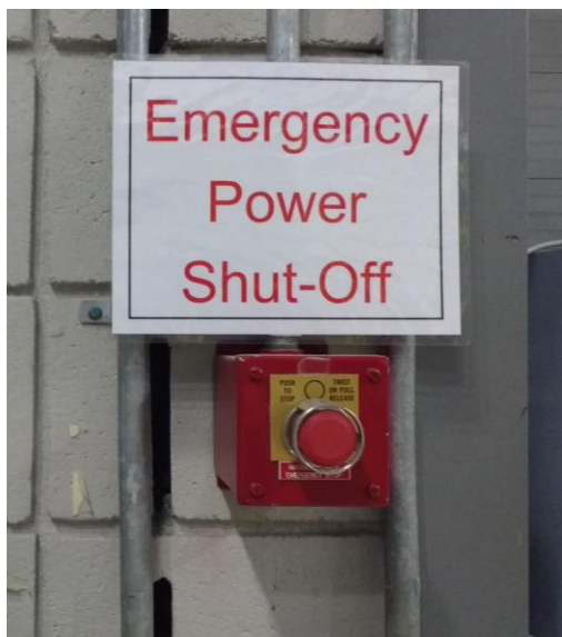
Figure 5: Emergency Power Shut-Off (EPO) button. These buttons are located on the wall close to the exit of the Magnet Cells.
