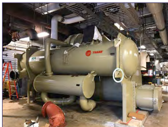
Figure 2.b.1: The first 7 MW (2,000 ton) chiller being installed.
